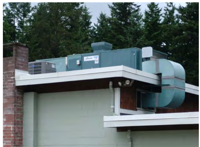
Figure 3 - LRGC Indoor Range heating and ventilation system mounted on the roof. This keeps the air clean and the range comfortable, especially in the winter.
