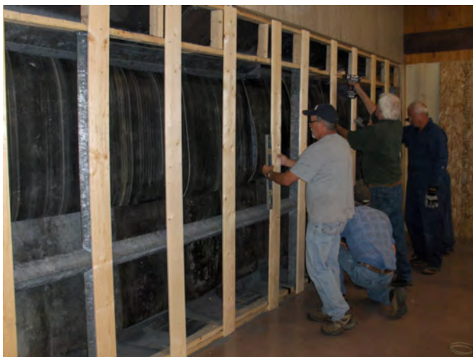
Figure 2 - This photo shows the conveyor belting covering the angled steel plating (look above conveyor belting) now visible with wood wall removed. Note that the steel plate stops at the 8 foot high mark - so keep your shots on the wood wall and NOT on the paneling above!
